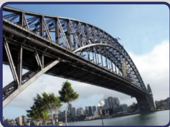
Sydney Harbour Bridge using Lindapter Fixings
