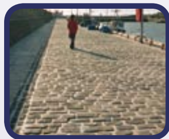
EasiPoint system with granite setts in Arbroath
