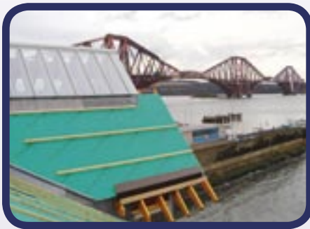
Proctor Roofshield membrane in Edinburgh
