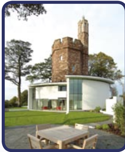
Lymm water Tower Conversion
