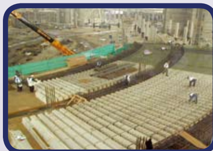
Cordek Formwork for the New Stadium in the Millennium Dome
